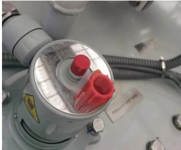
Figure 6-5 pressure relief valve safety cover
